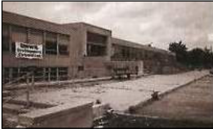
SESCO's Headquarters before Redevelopment
