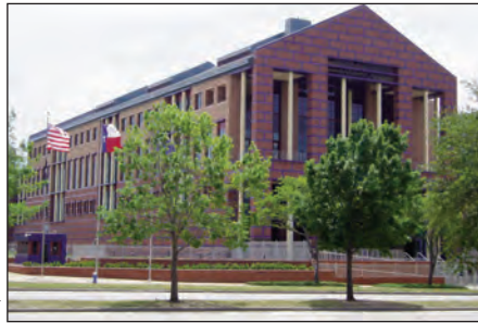
The Federal Reserve Bank of Dallas (FRBD) Houston Branch building located at a Brownfields site remediated using horizontal wells.
